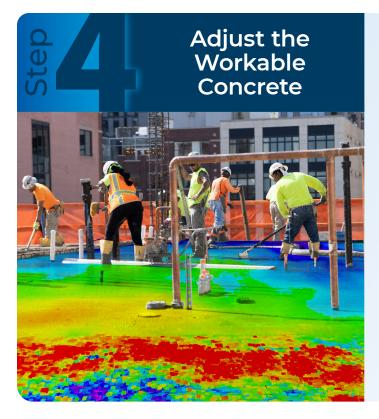
Thanks to the Flatness Check App, operators can easily identify – with pinpoint accuracy – any swells and dips in the concrete slab. Armed with this data, the team can perform the following tasks:
