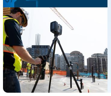
Set up the FARO Focus Premium Laser Scanner at the determined position. This can be accomplished manually or by driving the scanner via the Flatness Check app on iOS tablets, preferably a LiDARenabled tablet. (\*Note: Flatness Check still works with other iOS tablets) Select the appropriate resolution depending on the device's distance from the slab and perform the scan.
