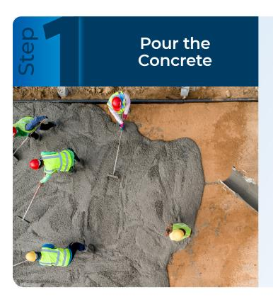
As the field crew prepares the job site and readies the concrete, those operating a laser scanner can determine where, and how many times, they will need to scan the slab. These pre-scan tasks can be performed before the concrete is poured, or while pouring/smoothing work is in progress.
